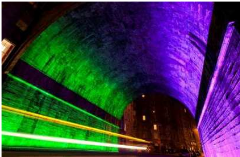
The Regent Bridge Edinburgh, UK
